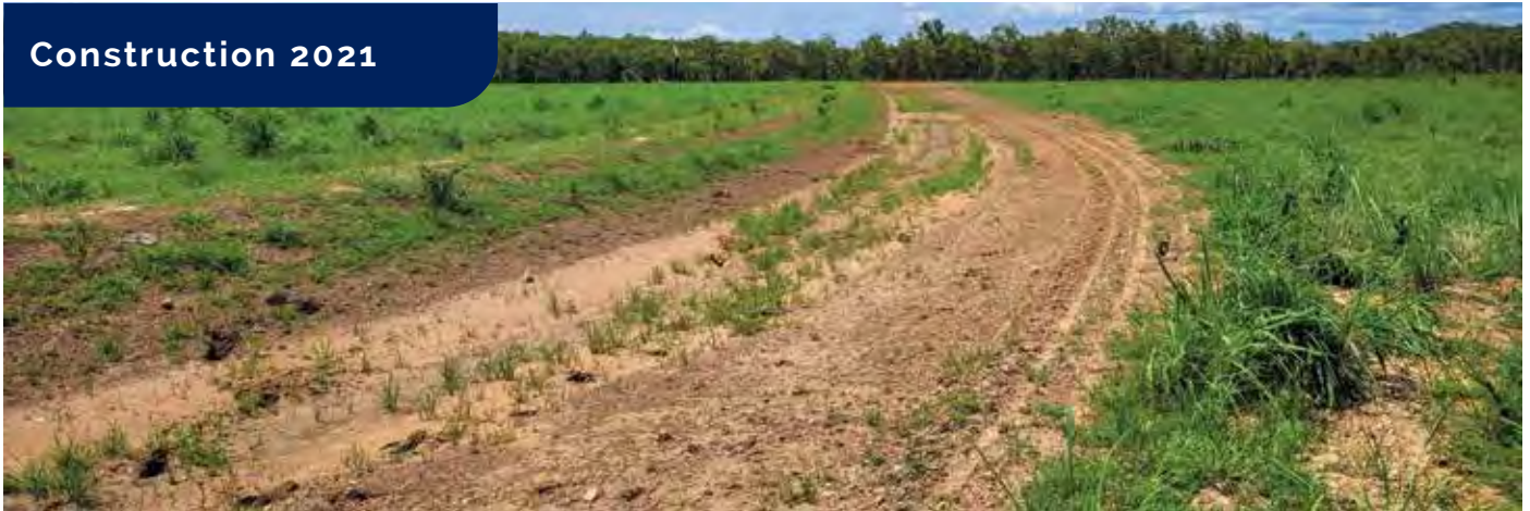
Old Cameron Downs Station Bachelor NT contour bank and swale with ponds at either end constructed in 2021 and after rainfall in February 2022 Credit: Fiona McBean landholder
