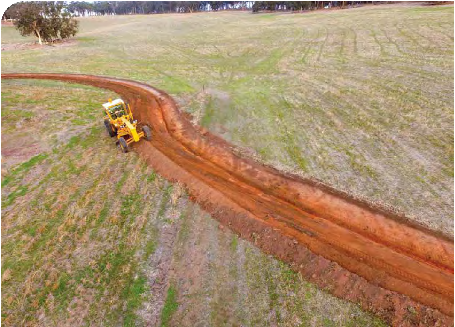
Contours being constructed at Paraway, Boyup Brook, WA in 2022. Credit:Lance Mudgway
