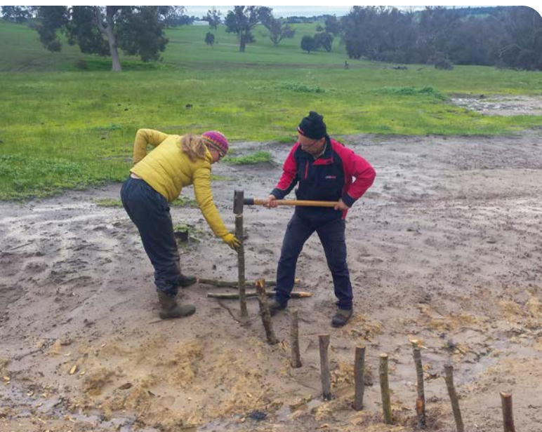
Above – Contour work completed, 2022
