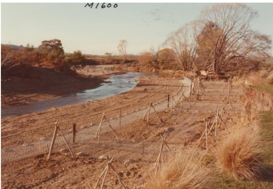
Figure 8 – One of many willow revetments constructed on the outside banks at Mulloon Creek between 1970 and 1980.
