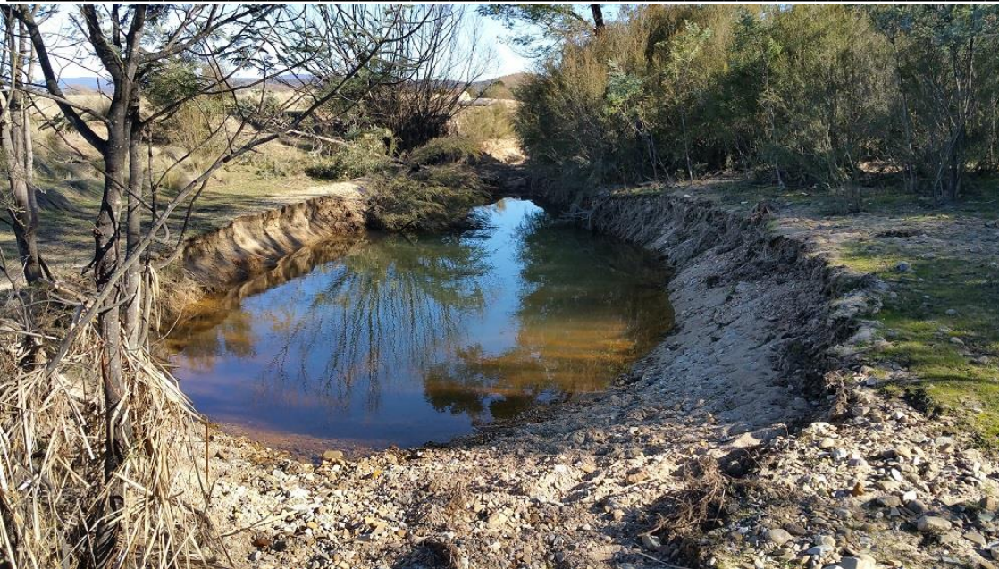
Figure 6 – Large hole blown in the secondary channel adjacent to MN1(2) and MN1(3) as a result of the June 2016 flood.
